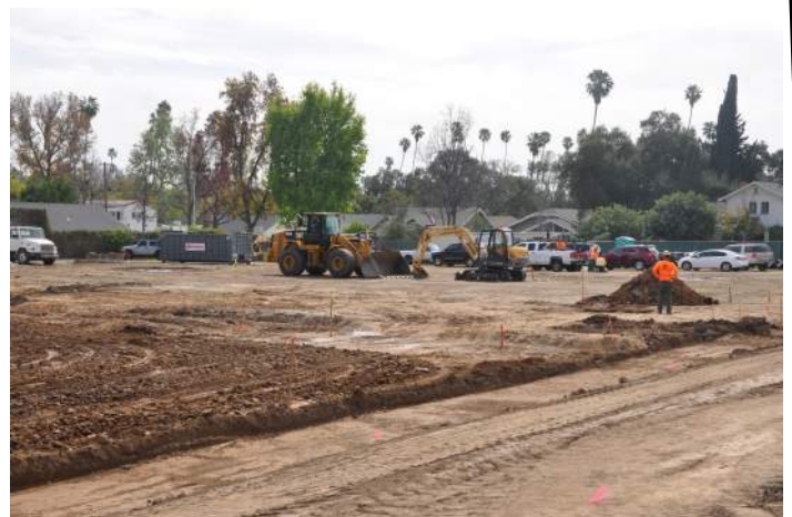
Middle School Hard Court & Field Project
