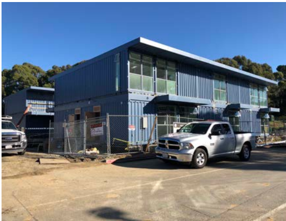
Buildings A and D are set
