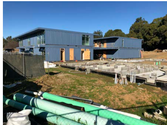
Ready for Building B first floor delivery on 2/24/2018
