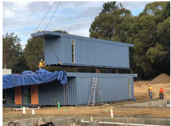
More modules being set, this completes Building D, and first Floor of Building A
