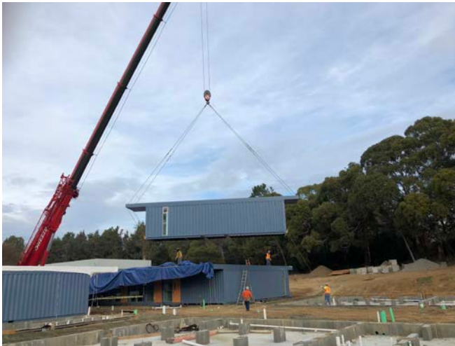
More modules being set, this completes Building D, and first Floor of Building A
