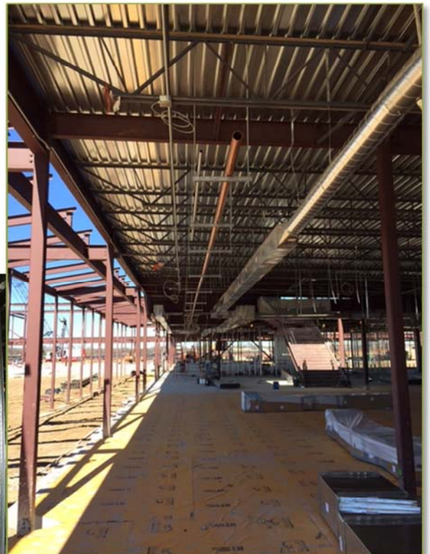
Interior metal studs and MEP above ceiling rough underway at classroom areas.
