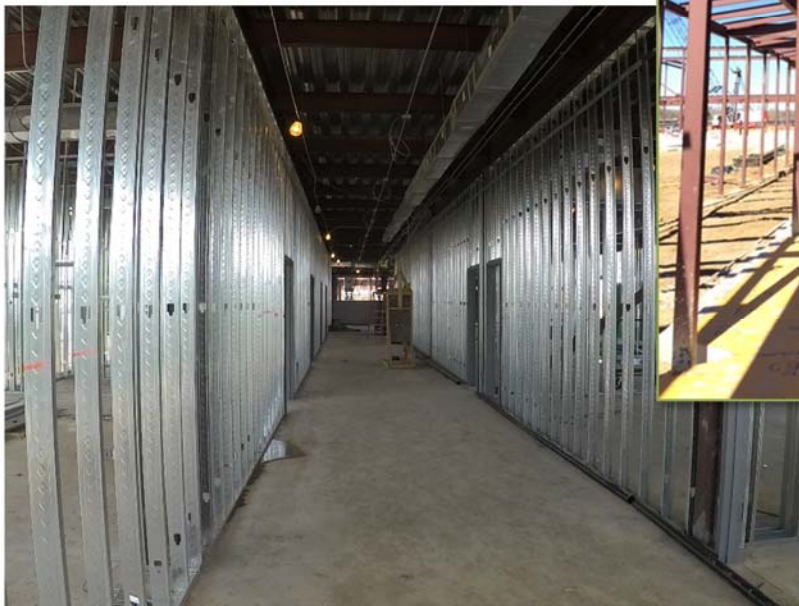
Interior metal studs and MEP above ceiling rough underway at classroom areas.
