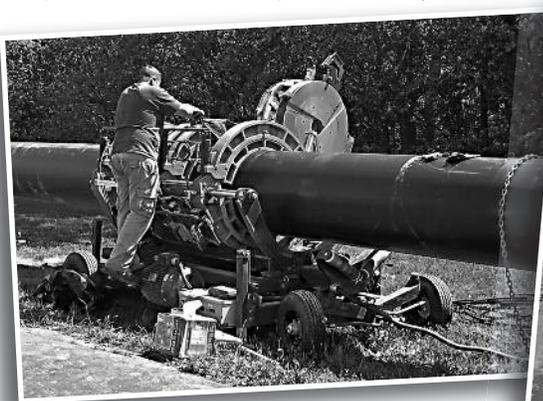
Water pipes were fused together under 480 pounds of pressure at 500 degrees F to create the pipeline that runs next to the septic field.
