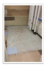
2 300 Wing Toilets: Remove existing fixtures, demolish existing CMU chase wall, Cut existing 24" deep concrete slab to remove imbedded existing fixture carriersexposed existing piping and start roughing new piping
