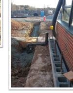
E2. Building "B" Addition: Under slab Radon Mitigation/ Plumbing pipe installation, Concrete slab preparations
