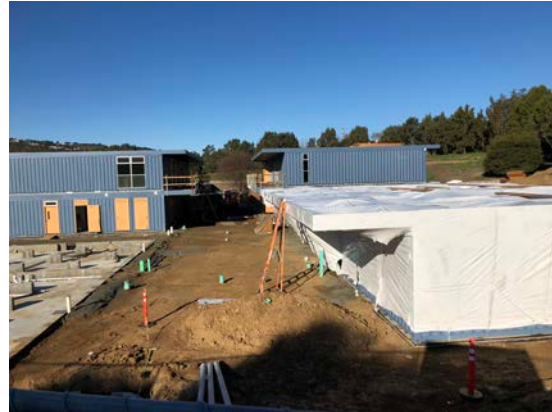
Buildings A and D are set
