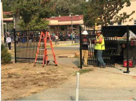
New fencing at Tierra Linda
