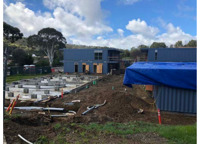
Buildings A and D are set
