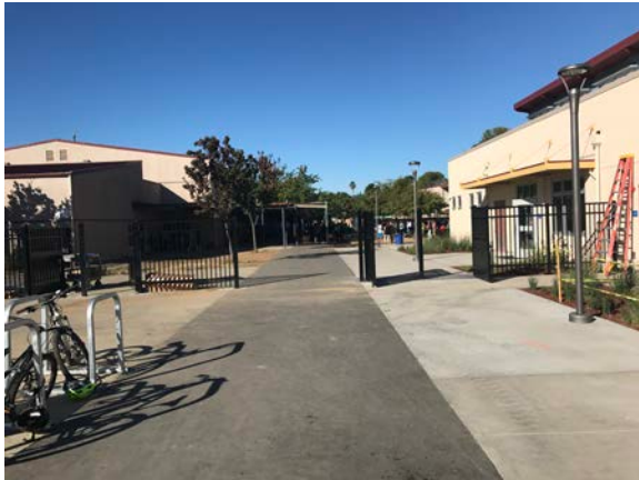
New Fencing at Tierra Linda
