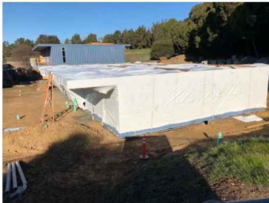
Building B first floor on site and weatherproofed
