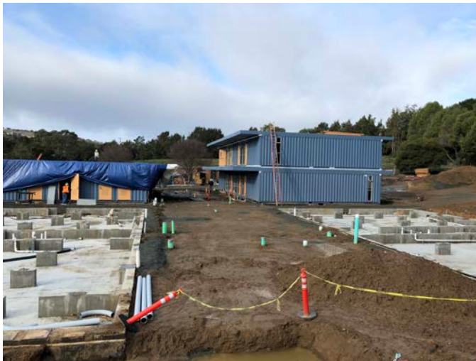
Buildings A and D
