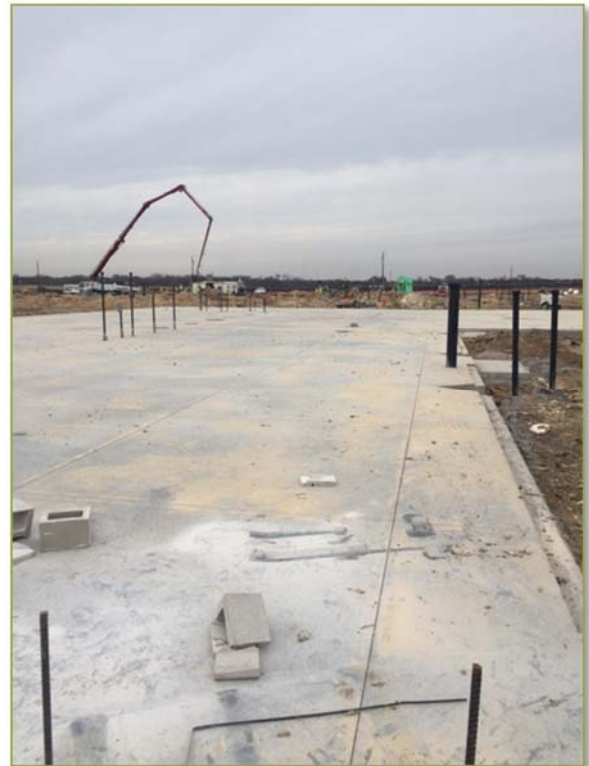
Setting steel at the Auditorium, slab poured at Area "E" (Classrooms) and CMU underway at Area "J" (Black Box and Band Area).
