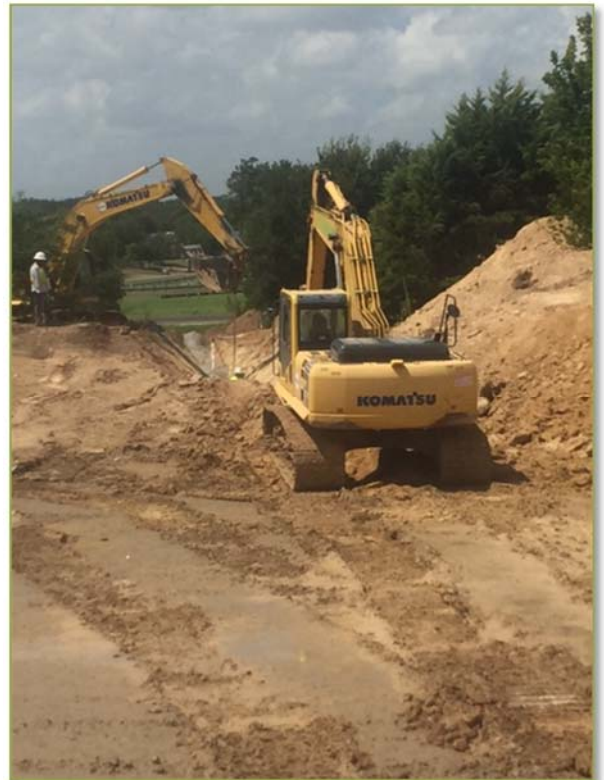
Starting installation of main water line – north to south along the main ring road. Installing underground storm line along the west side of property.
