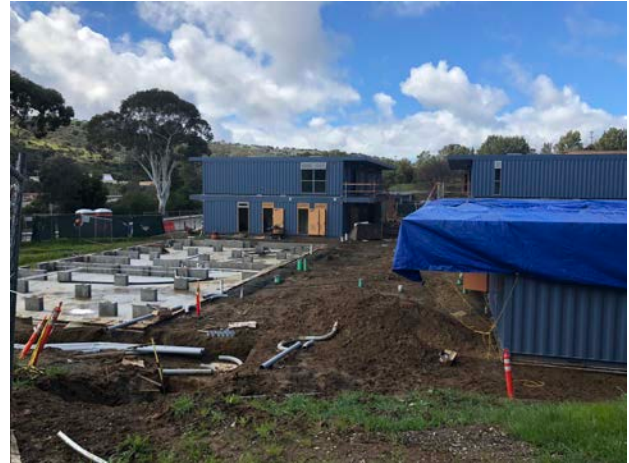
Buildings A and D are set
