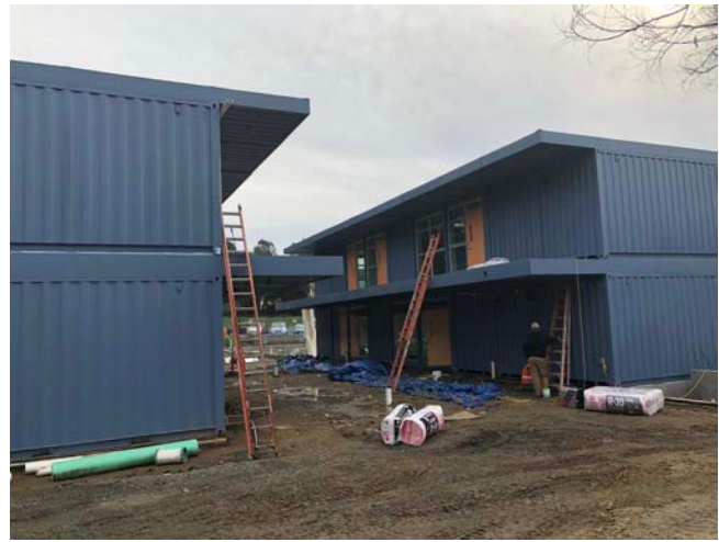
Buildings A and D in place
