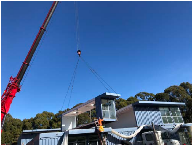
Building D second floor being set
