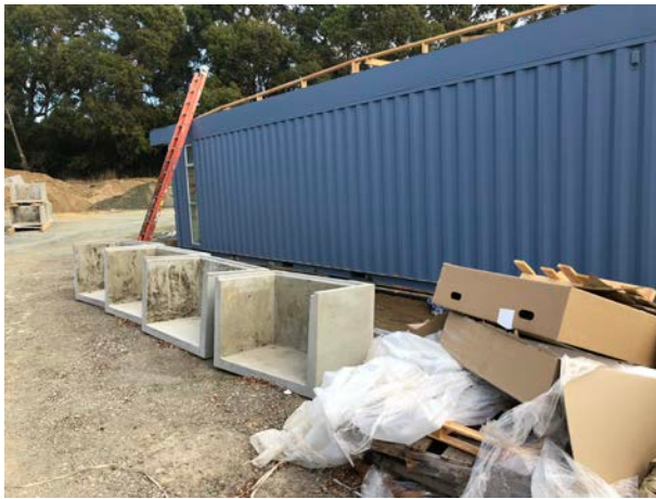
Pre-Cast Wells - Foundation Vents
