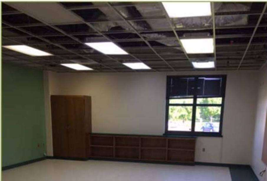
Ceiling tiles missing due to installation of fire suppression system, campus wide.
