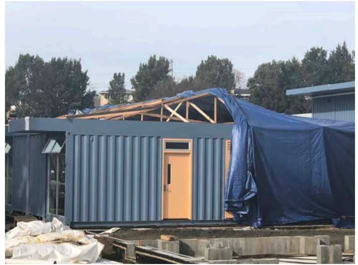
Building D - working around weather protection, making preparations for second floor delivery
