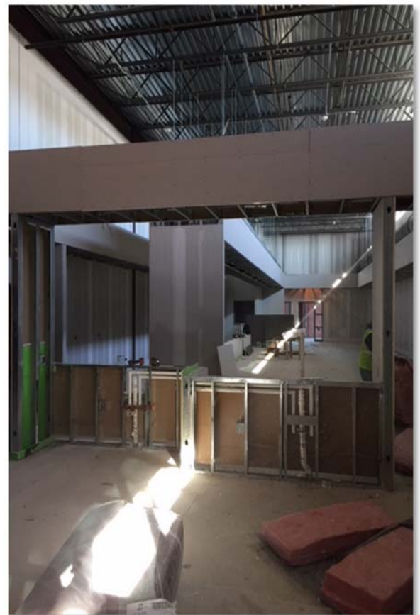
Sheetrock and tape and bed, storefront installation ongoing in CTE area
