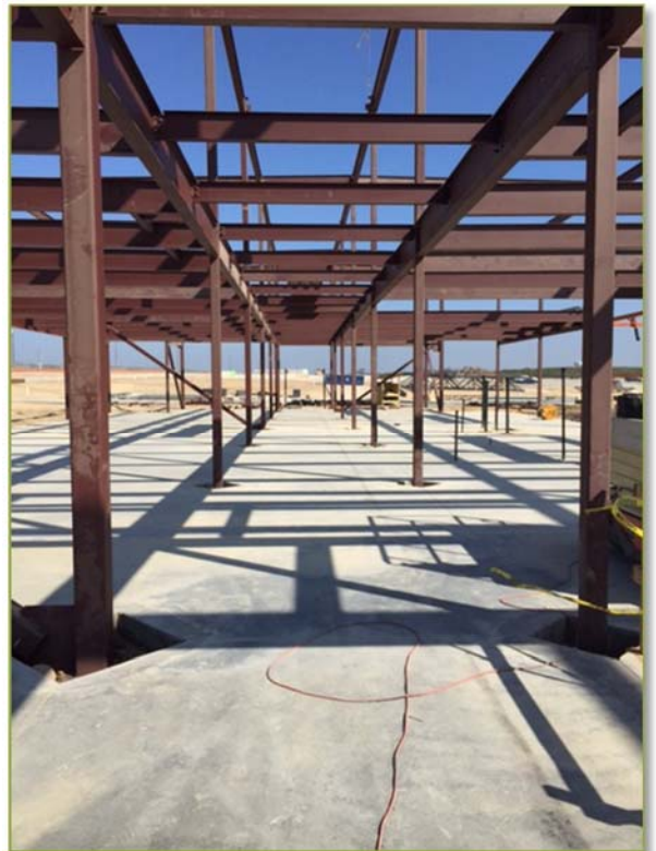
Hanging steel and exterior metal studs at classrooms wings.
