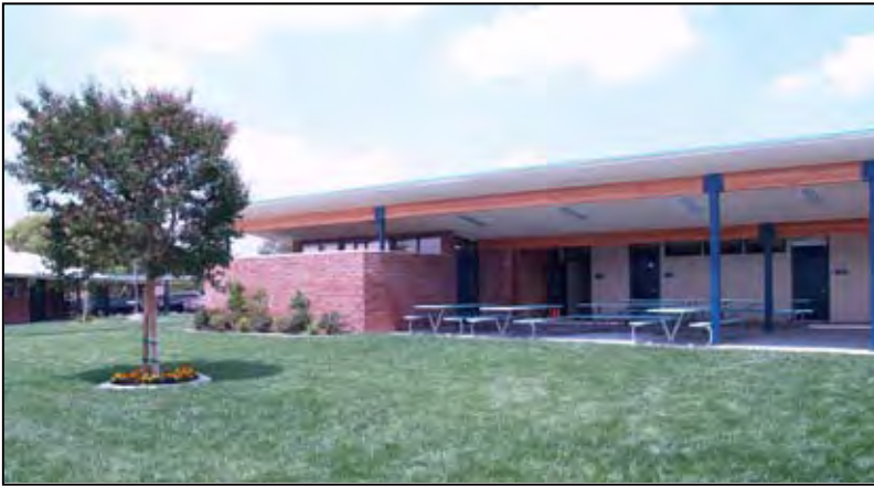
New Multipurpose Room, Staff Lounge and Teacher Prep Area.
