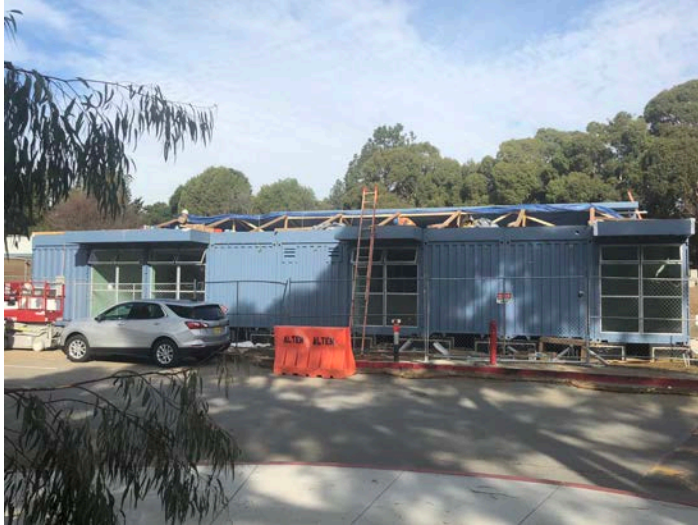
Building A - working around weather protection, making preparations for second floor delivery
