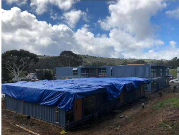
Building B first floor on site, weatherproofed, ready to weld and secure
